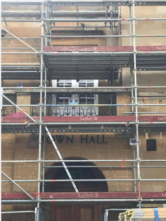
External Works on the Town Hall Start – August, 2021
